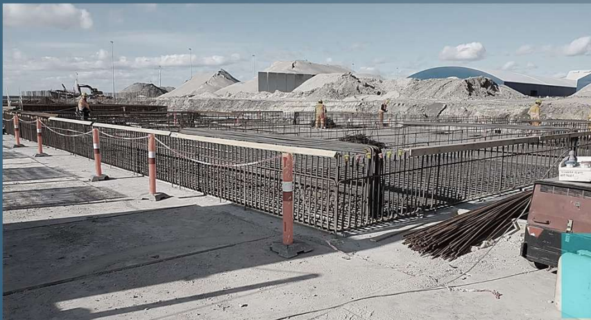
FOUNDATION STEEL BARS POSITIONING FLOOR CASTING OF PREFABICATION CAMP
