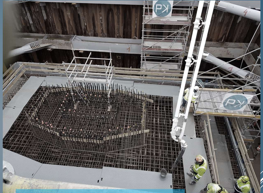
FOUNDATION STEEL BARS POSITIONING PILES N. 22-23 SOUTH
